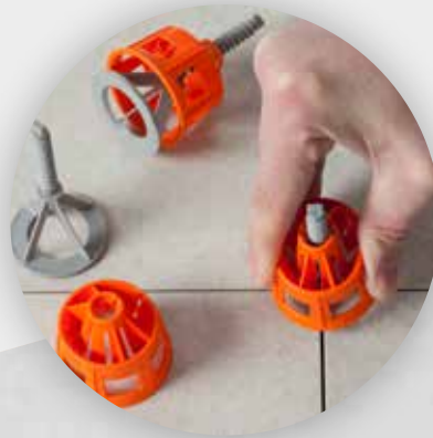
PLACE THE PIECE WITH YOUR HAND AND SCREW IN
