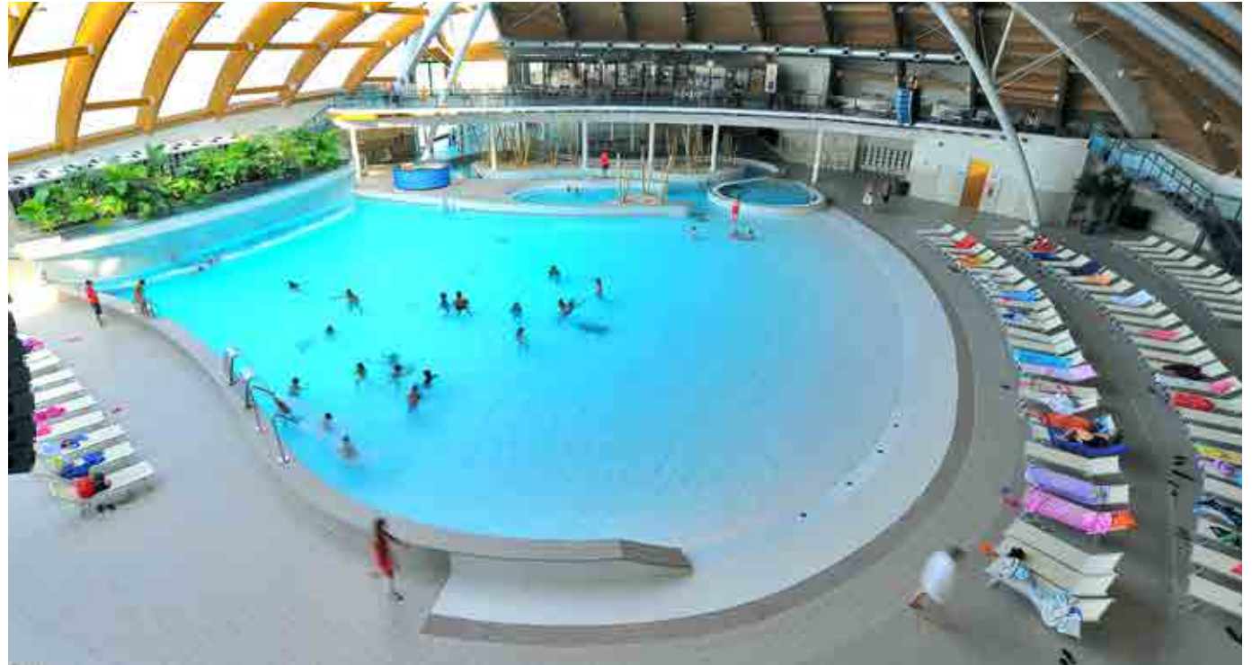
Aquaworld | Concorezzo, Italy | Architect: Federico Pella
