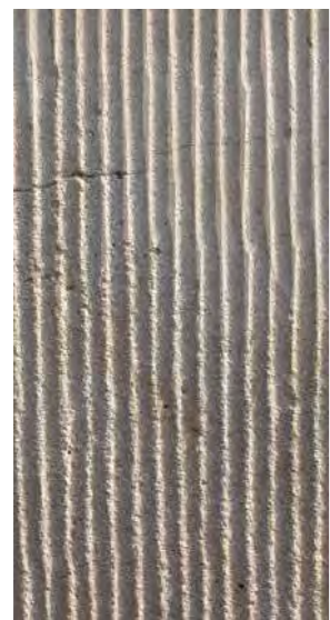
Detail of a wall, Vindebrogade
